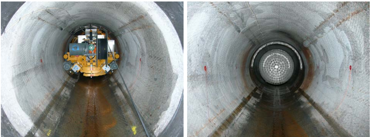
Figure 4-3. (left) The deposition machine inside the 95 m long drift at -220 m level at Äspö HRL (right) The perforated end plate of the Supercontainer in the same drift.
