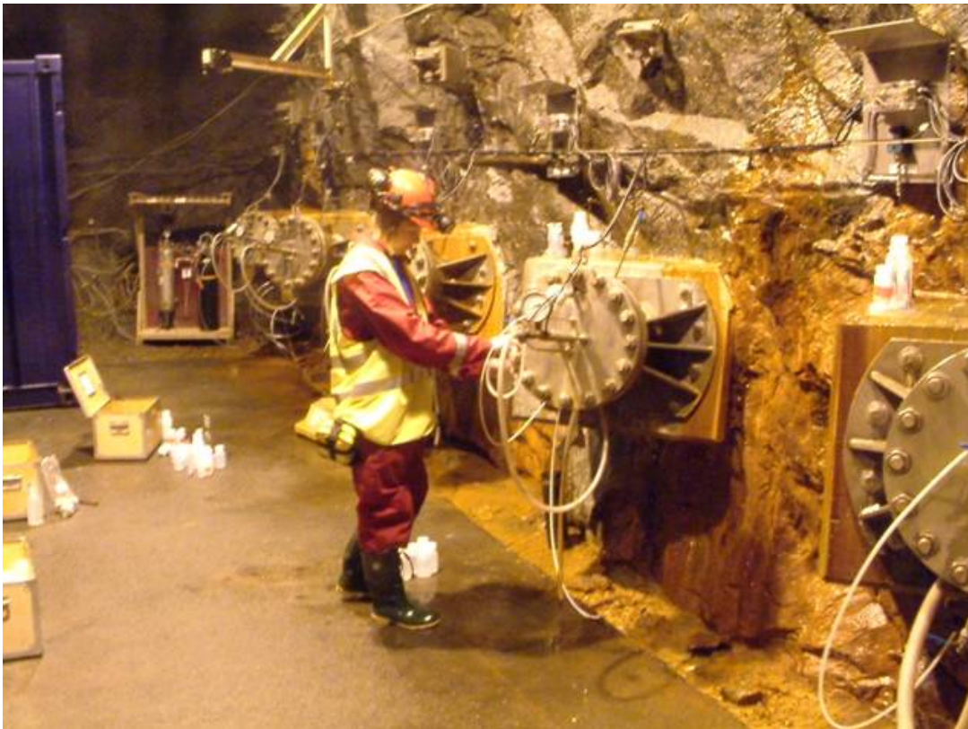
Figure 4-1. The installation of the In Situ Corrosion Testing of Miniature Canisters.
