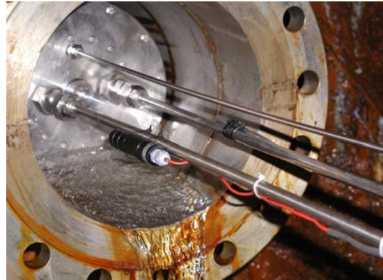
Installation of first model canister assembly
